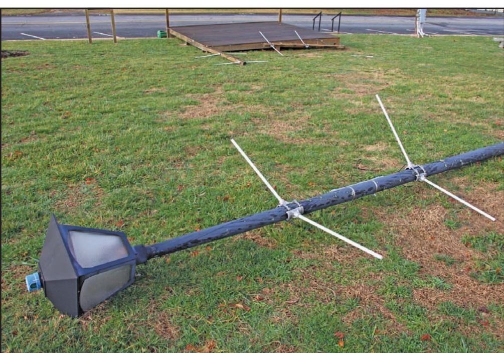
The Hiawassee Town Square suffered some wind damage Saturday, including this downed light pole and some stage damage. Photo by Shawn Jarrard
